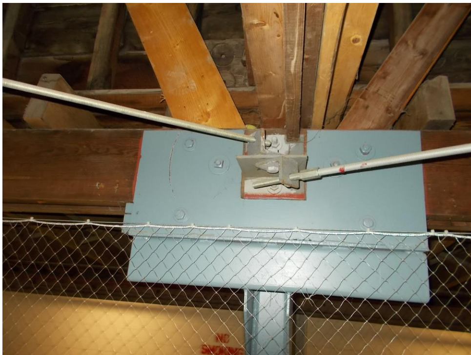
Reinforcing at steel columns
