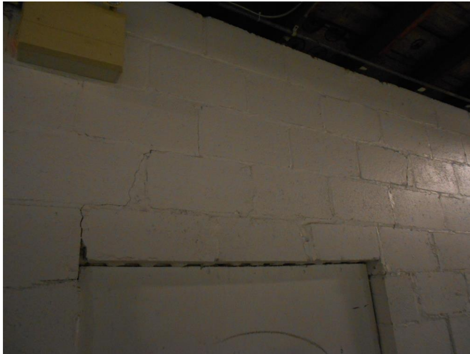
Step cracking in exterior block
