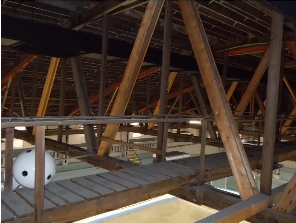
Catwalk between trusses
