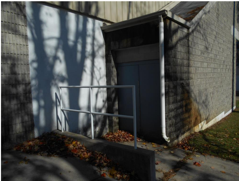
Black staining on block at south stair
