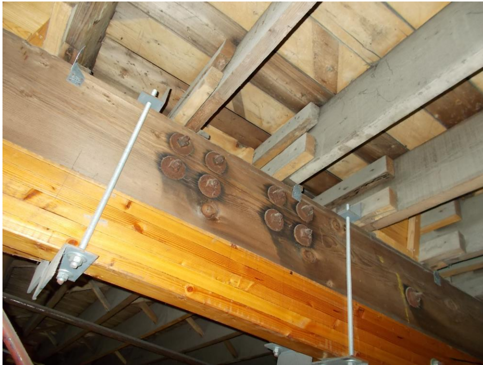
Reinforcing of trusses
