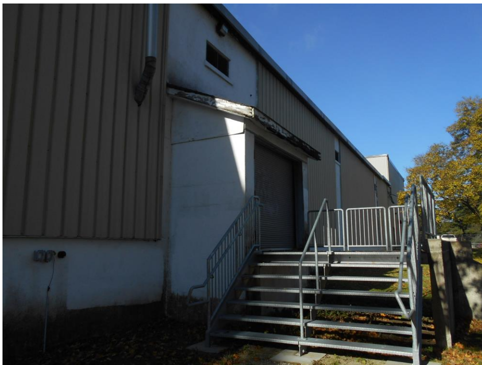
Covered extension on east should be replaced
