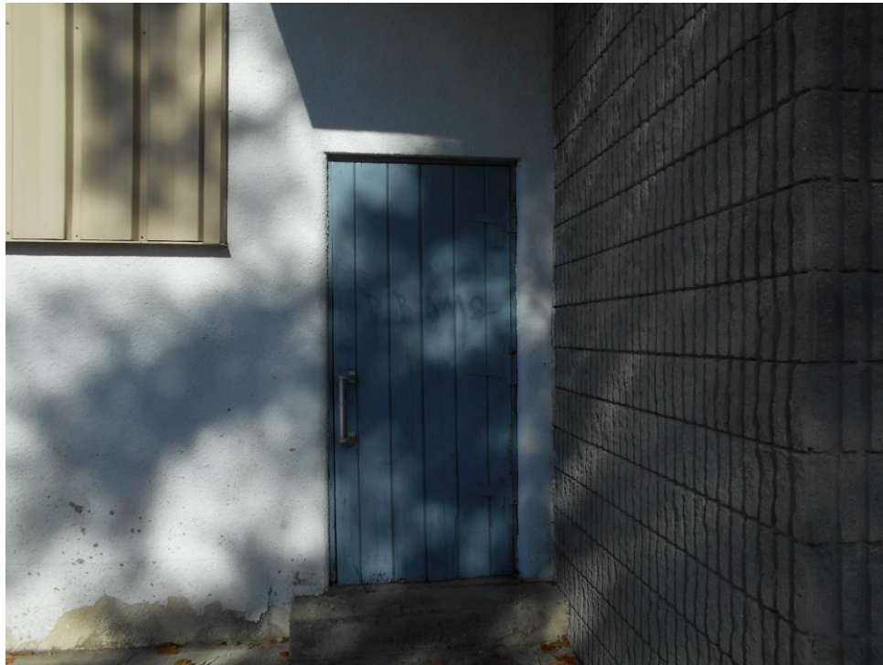
Old wooden door to be replaced, damaged stucco
