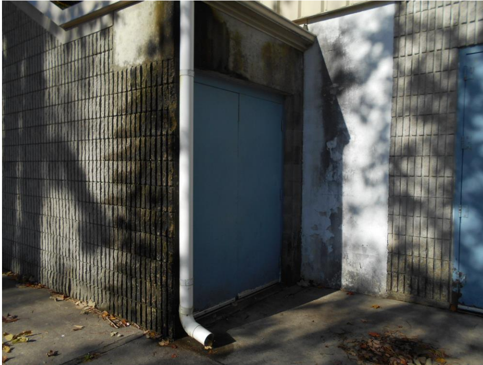
Black staining on block at south stair and along top at roof, damaged stucco
