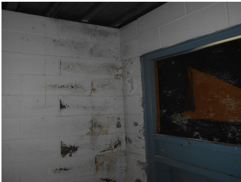
Moisture on interior walls south end
