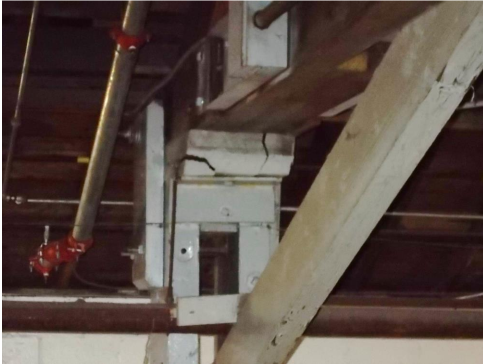
Cracked bolster block
