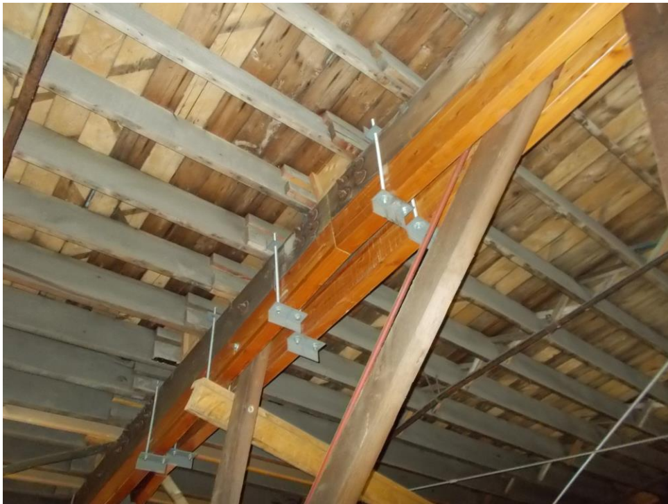
Reinforcing of wood bow truss.
