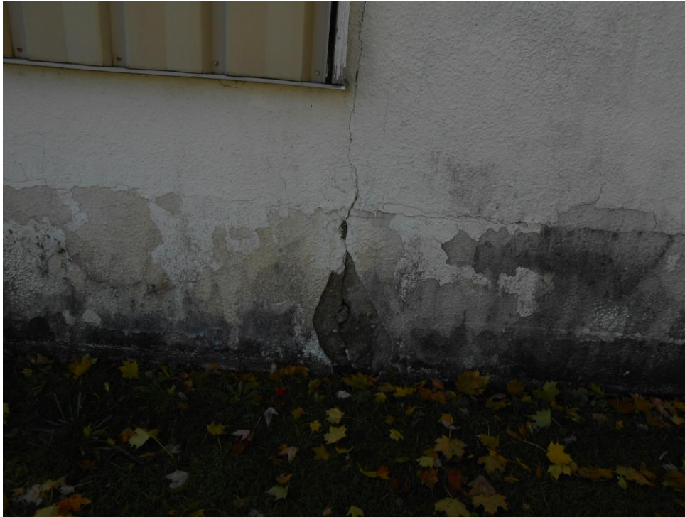
Cracked stucco and foundation on east side
