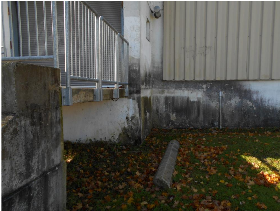
Damp, black staining on exterior walls at east exit
