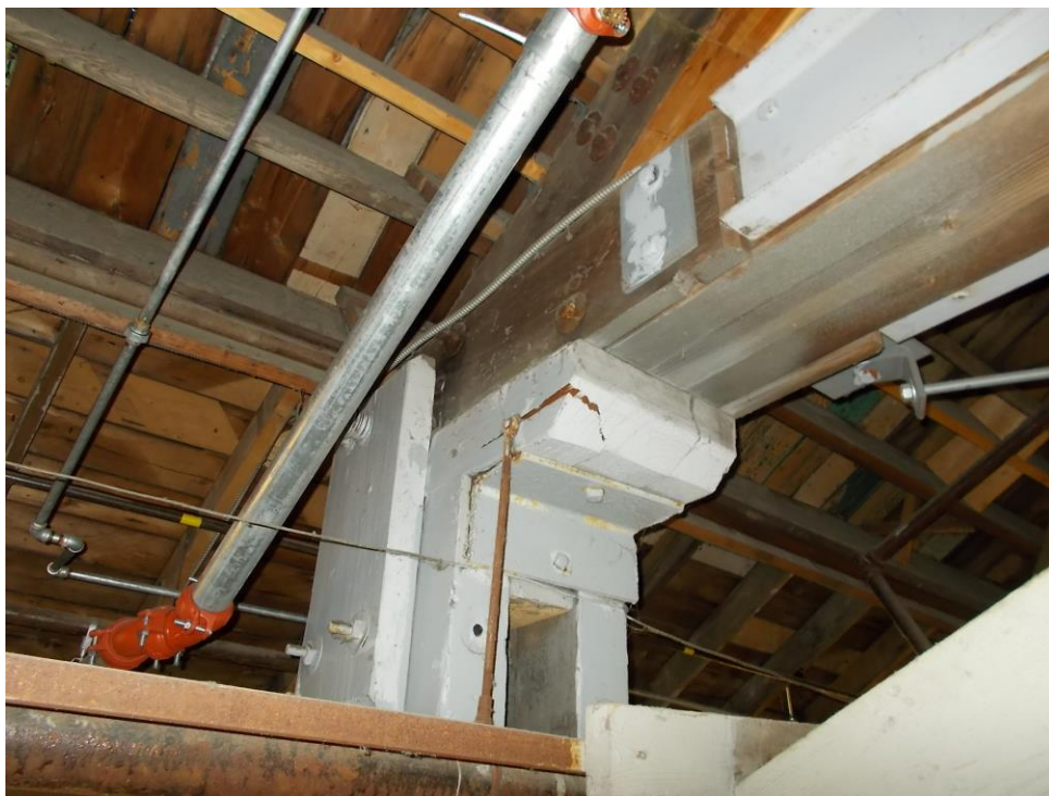
Cracked bolster block
