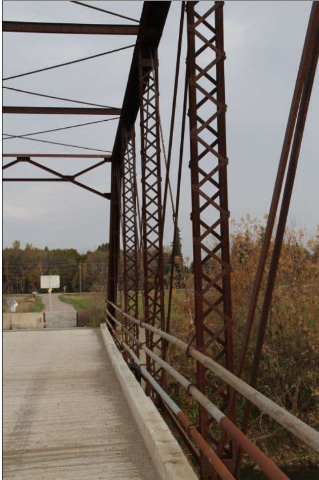
Figure 29 steel rod diagonal members & sway bracing
