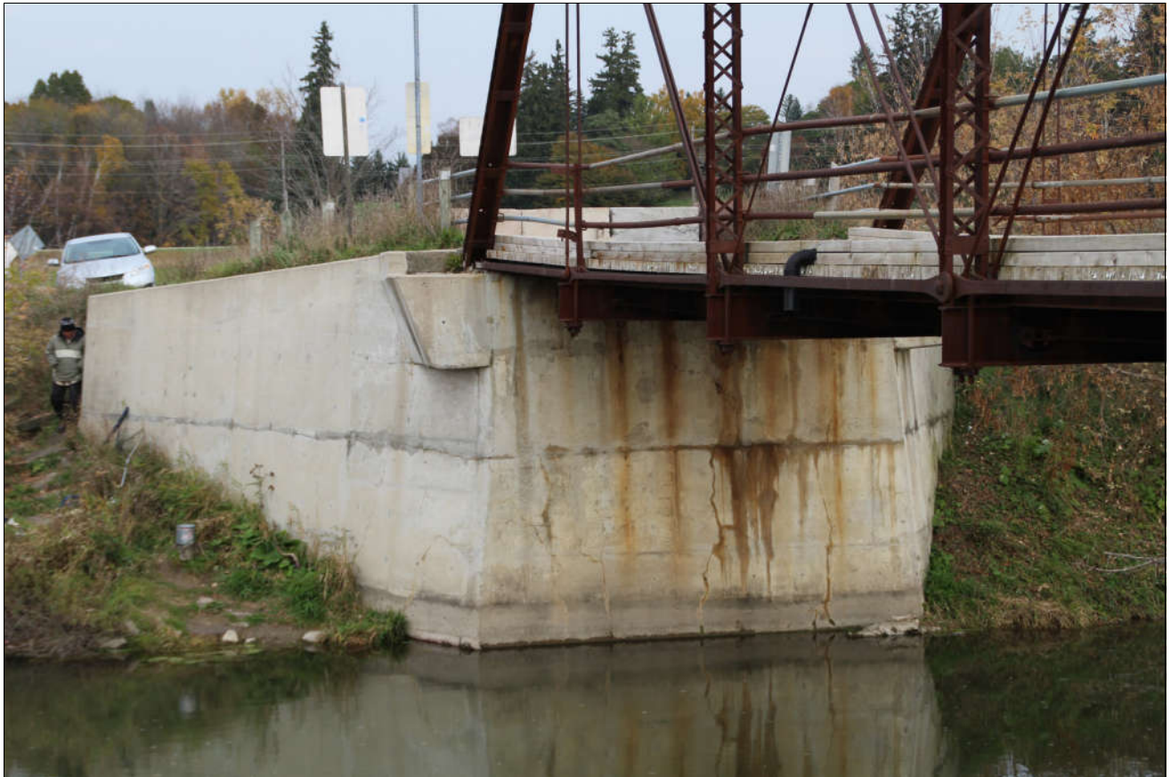
Figure 41 north abutment - visible sag in bridge bottom chord
