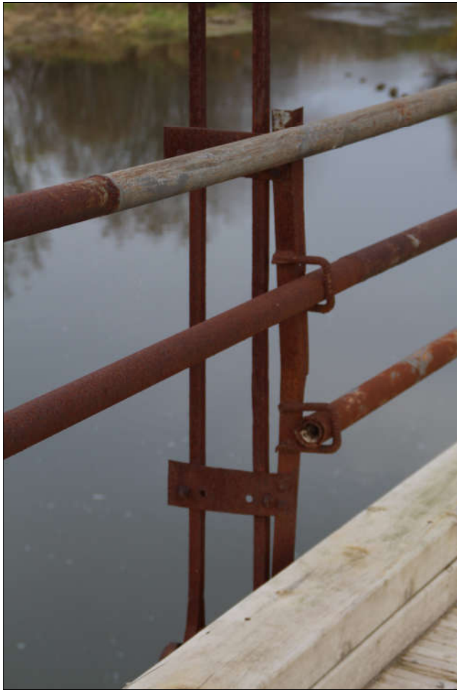
Figure 33 pipe railing with missing section
