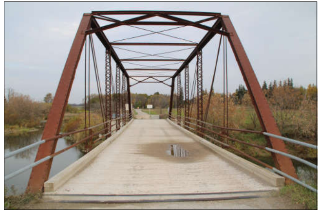
Figure 34 bridge deck - note ponding near southeast end
