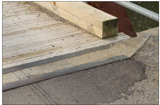
Figure 35 bridge deck, curb & expansion joint
