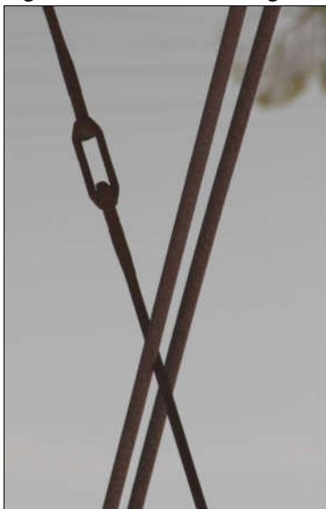
Figure 31 turnbuckle
