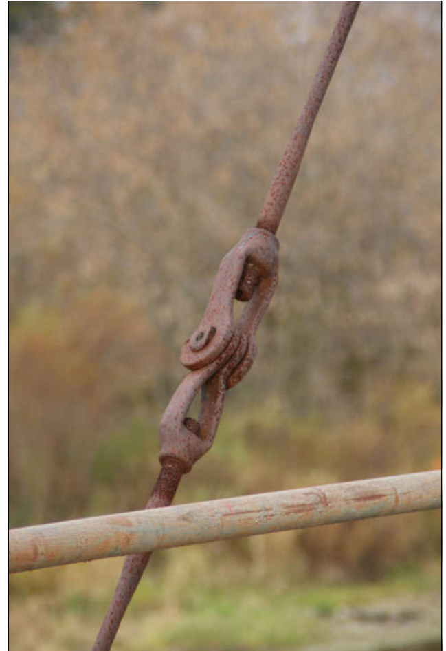
Figure 30 unusual turnbuckle
