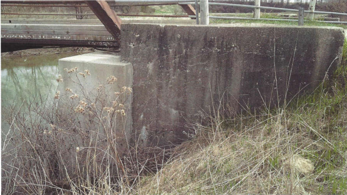
13. Southwest Wingwall - Cracking with Efflorescence
