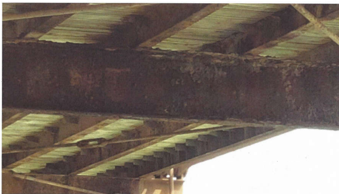
16. Second Beam from South - Severe Corrosion with Perforations
