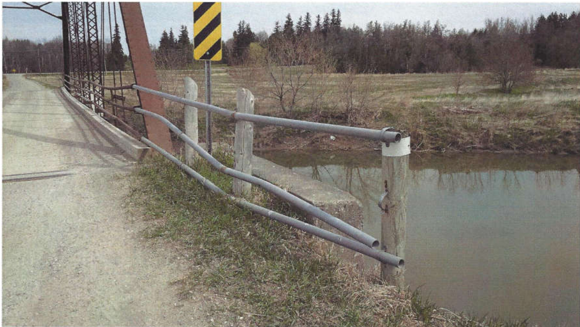
7. Approach Barrier at Southeast - Impact Damage
