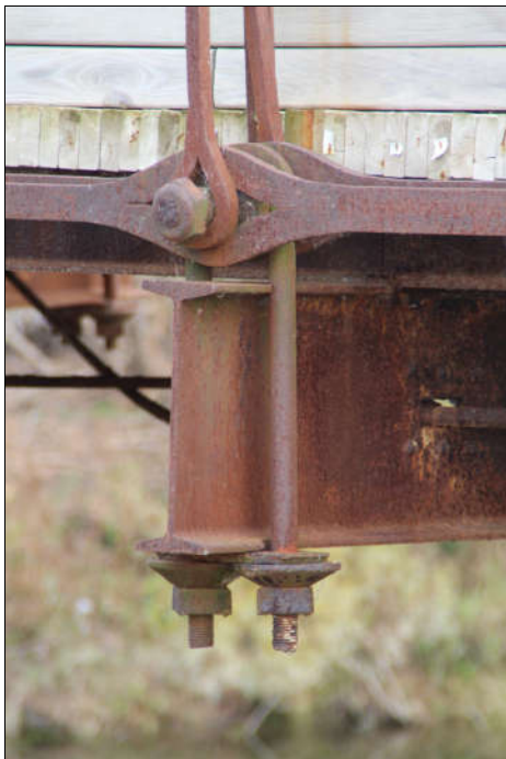
Figure 27 bottom chord/beam connection
