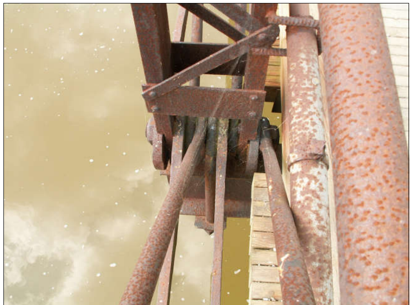
Figure 28 bottom chord connection - historicbridges.org
