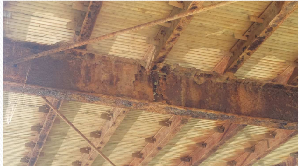
Severely Deteriorated Floor Beam
