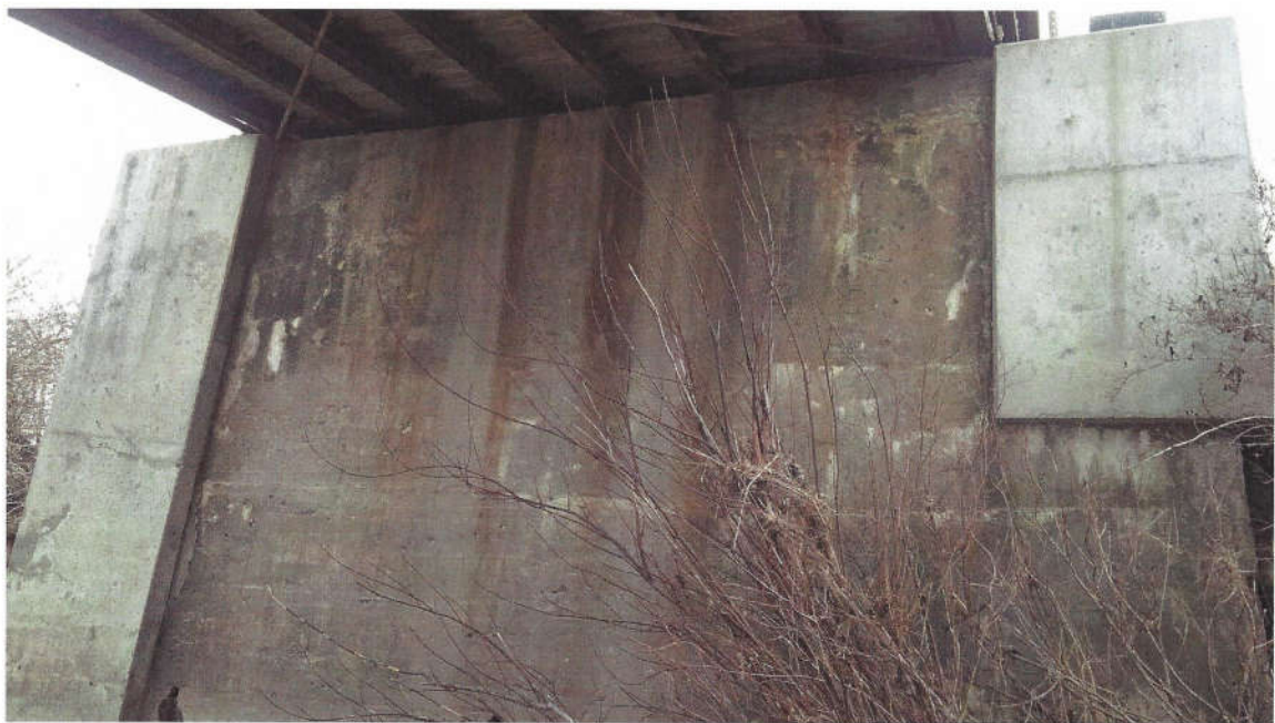
12. South Abutment - Cracking with Efflorescence
