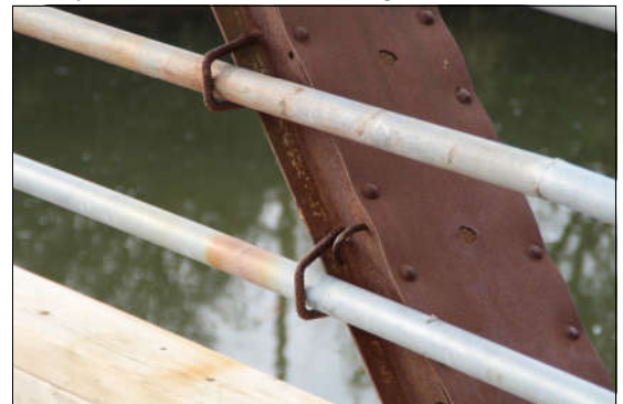
Figure 32 pipe railing connection to end post
