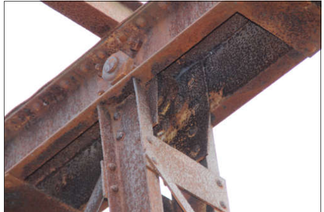
Figure 25 top chord pinned connection and batten
