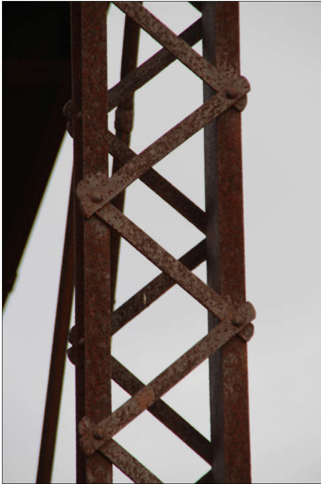
Figure 24 V-laced vertical member
