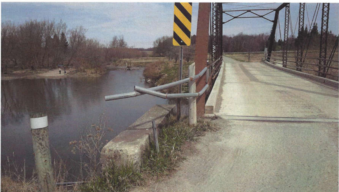
8. Approach Barrier at Southwest - Impact Damage
