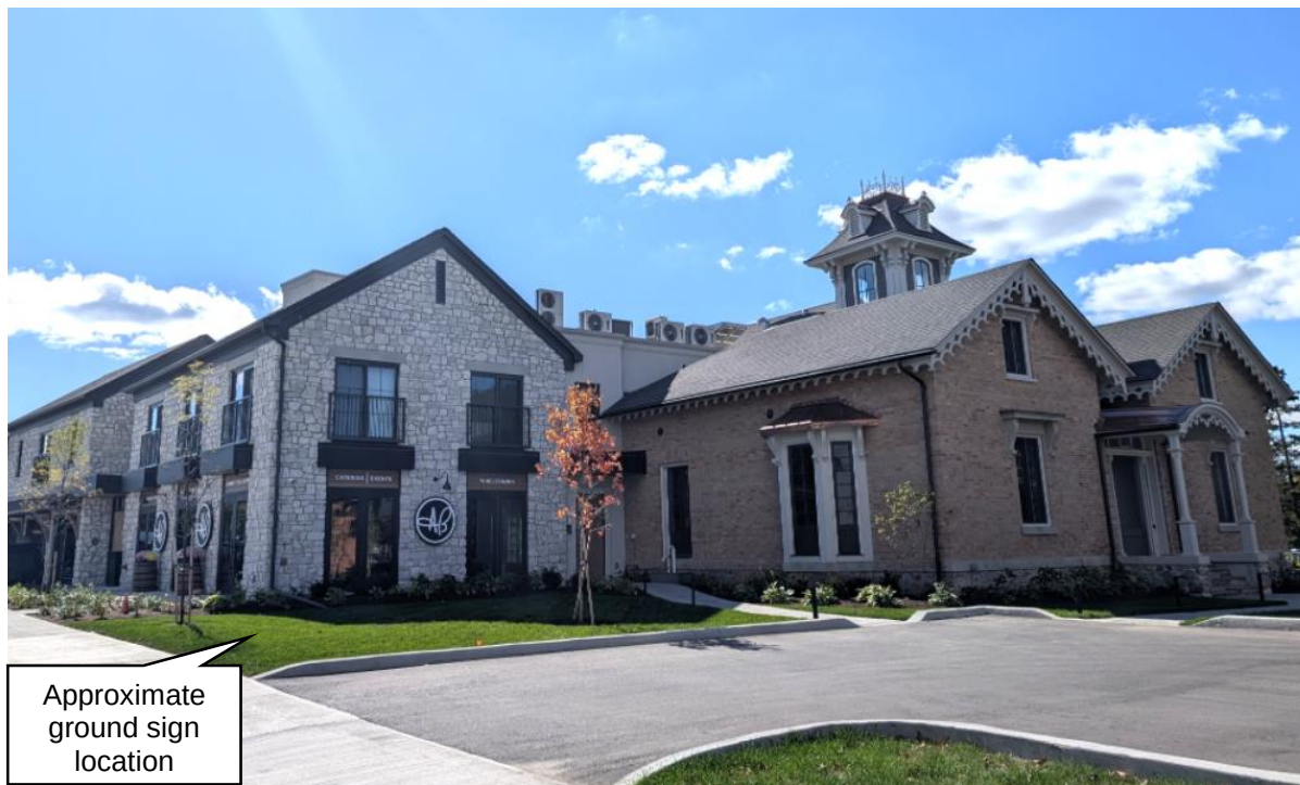
Figure 4 Front/Side Facade of the Waterlot facing South on Wilmot Street
