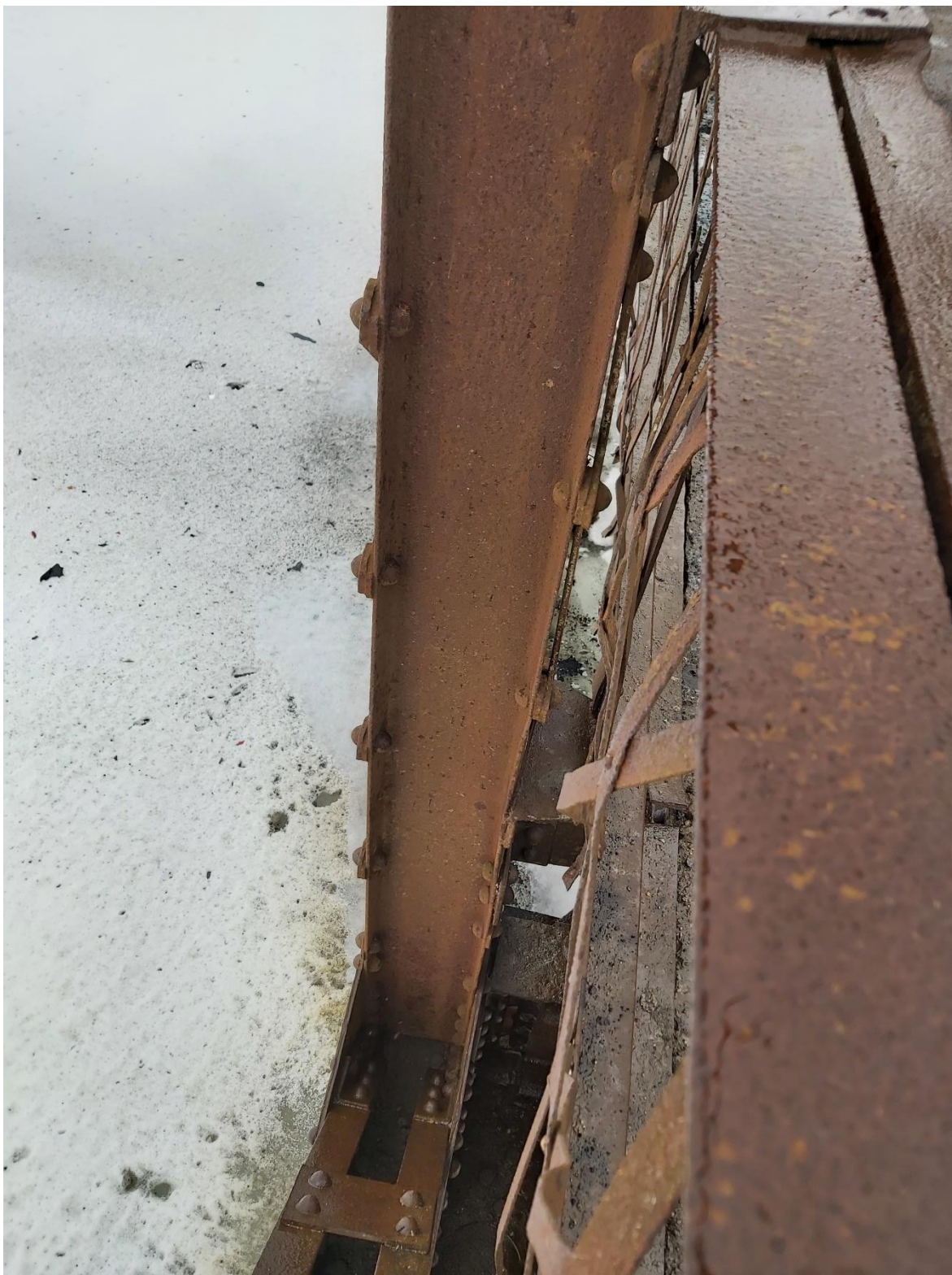
North side, fifth vertical from east end – minor deformation of vertical member from impact
