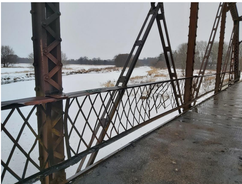
North Side, fourth bay from east end – heavy damage to railing panels. Also note blackened area at deck and structural members.
