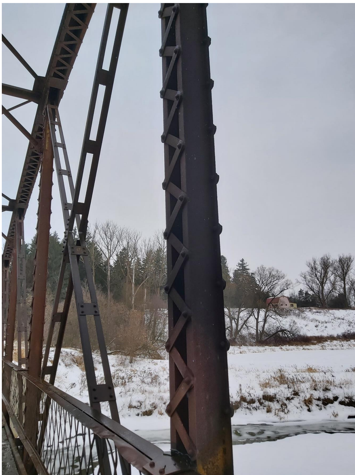
North side, fourth vertical from east end – note blackened areas from vehicle fire
