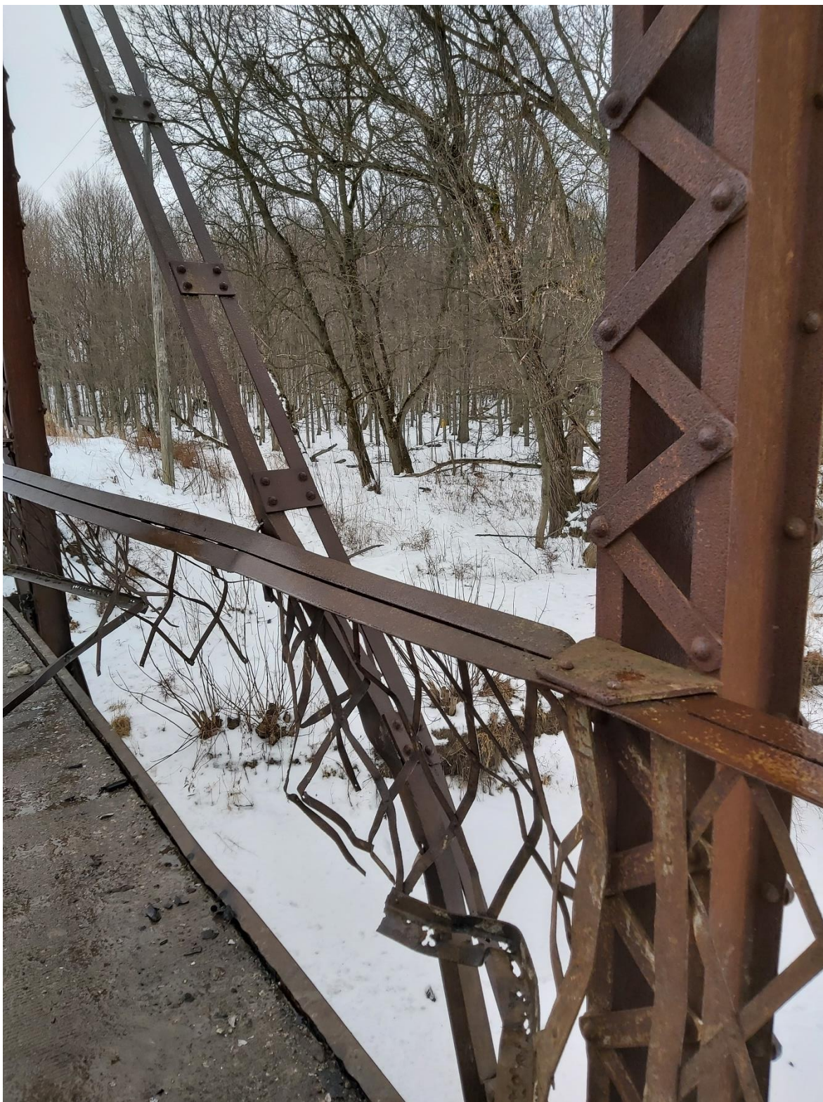
South Side, third bay from east end - Severe damage at railing panel and diagonal structural member.
