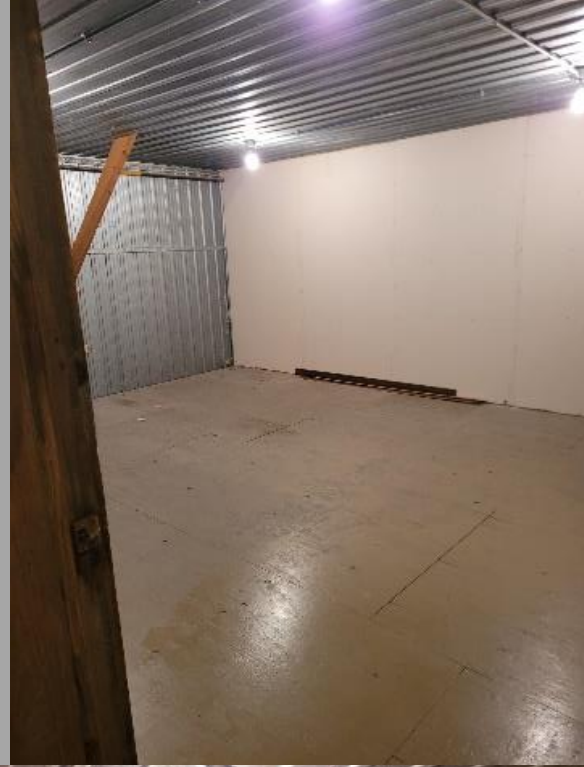
Second Floor Archive/Storage Room
